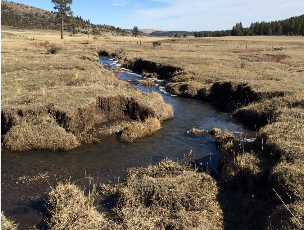
Figure 6 An erosional bank with a fracture feature and slump blocks below the scour line. (Renner, et al., 2023)
