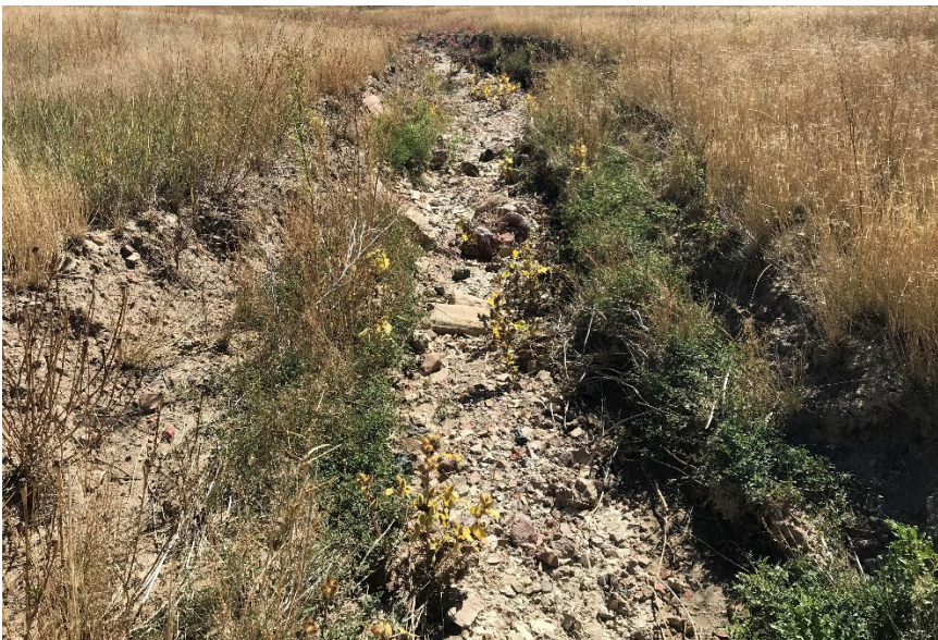
Figure 8. Transect R2 of the reclaimed drainage. Stability analysis classifies this reach as potentially stabilizing.
